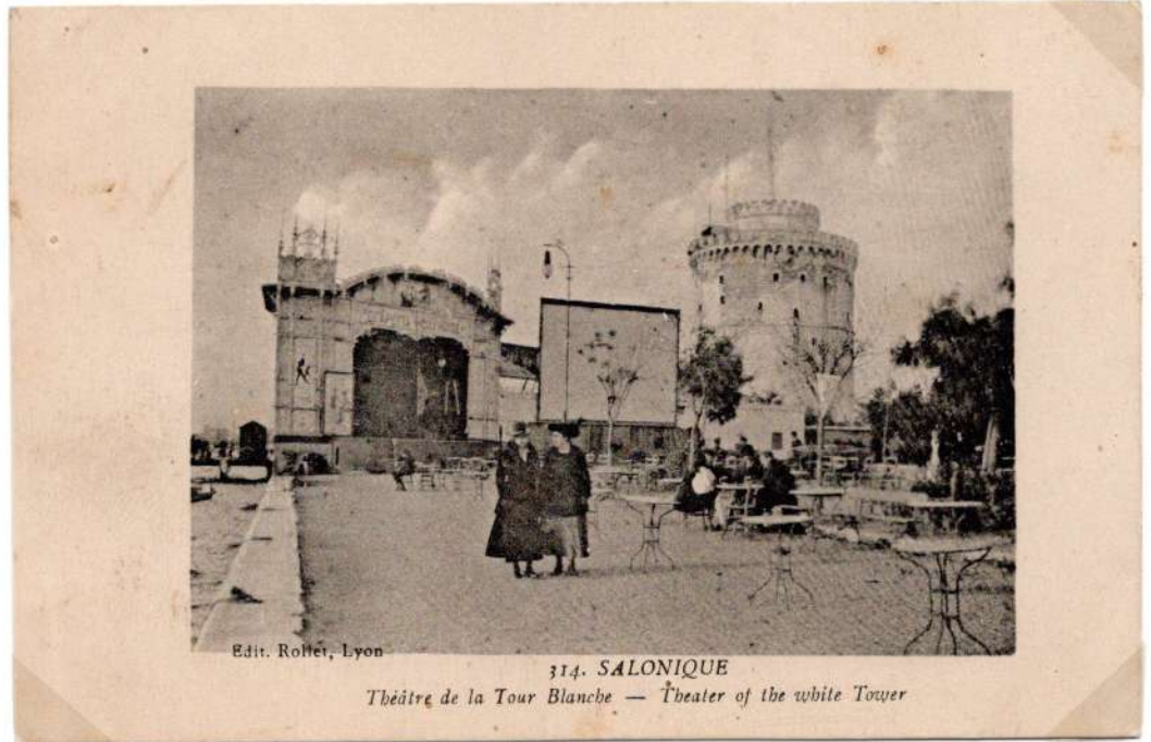
The White Tower Theater. On the left, the Thermaïcos Gulf.
